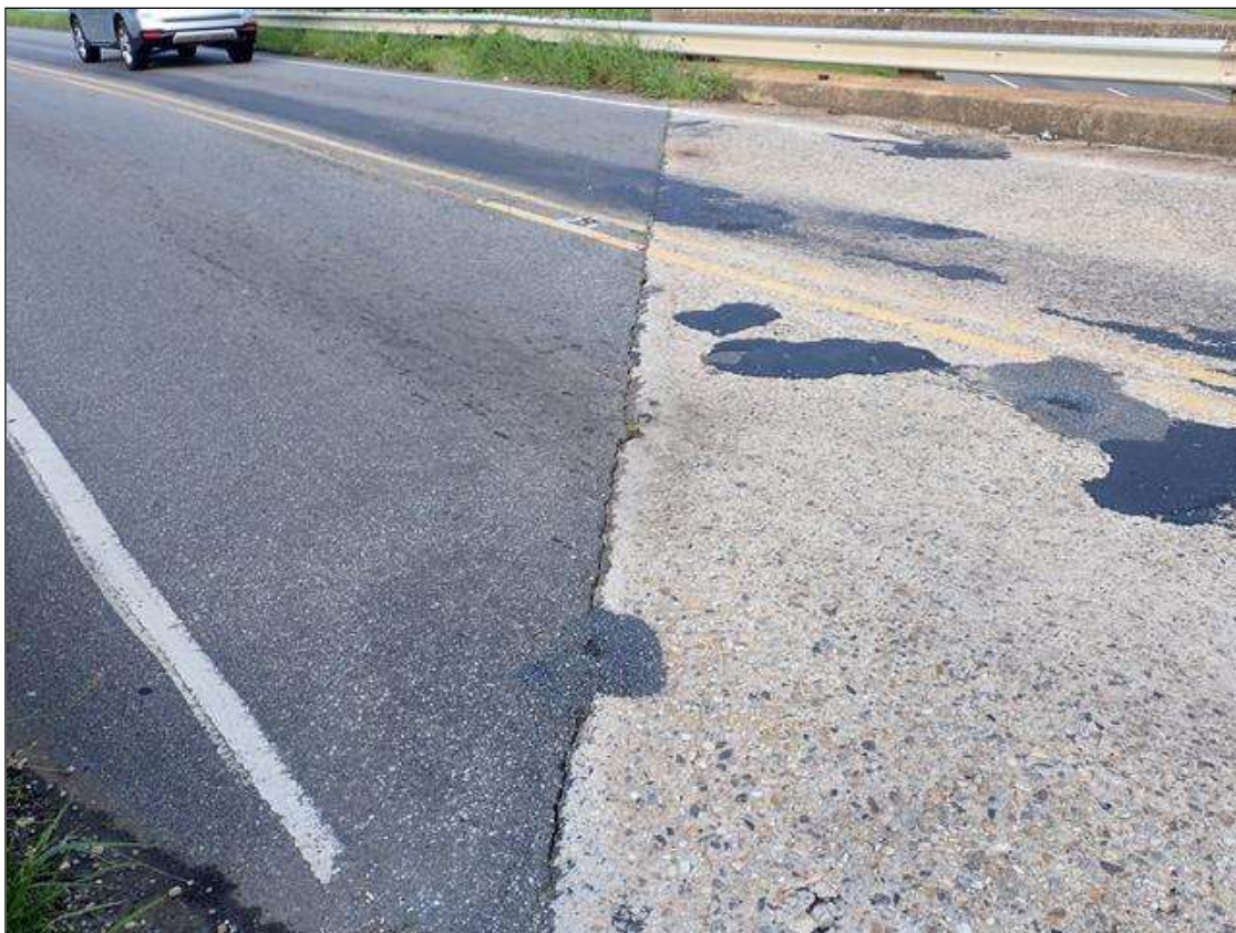
end bent 1 deck
