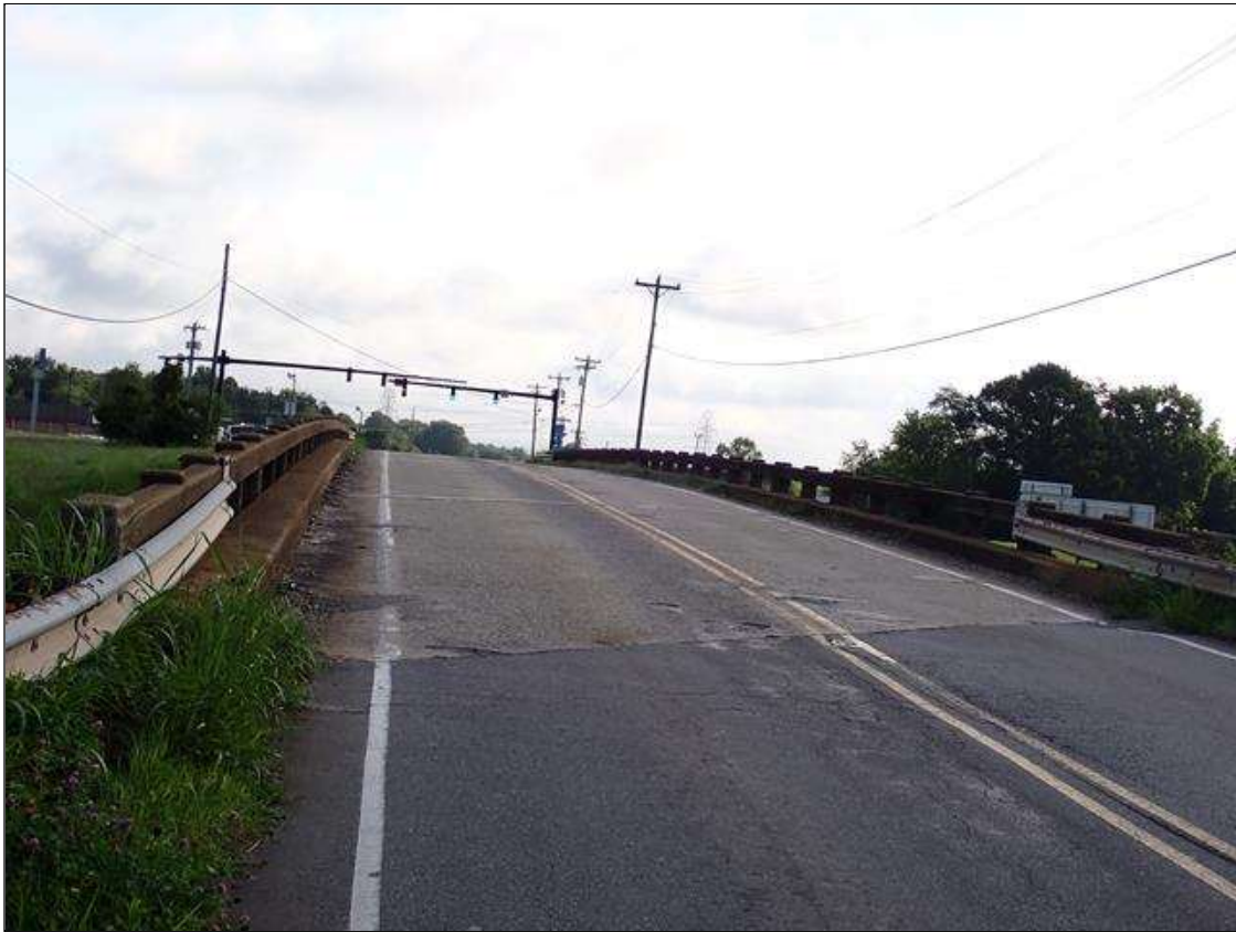
south approach looking north
