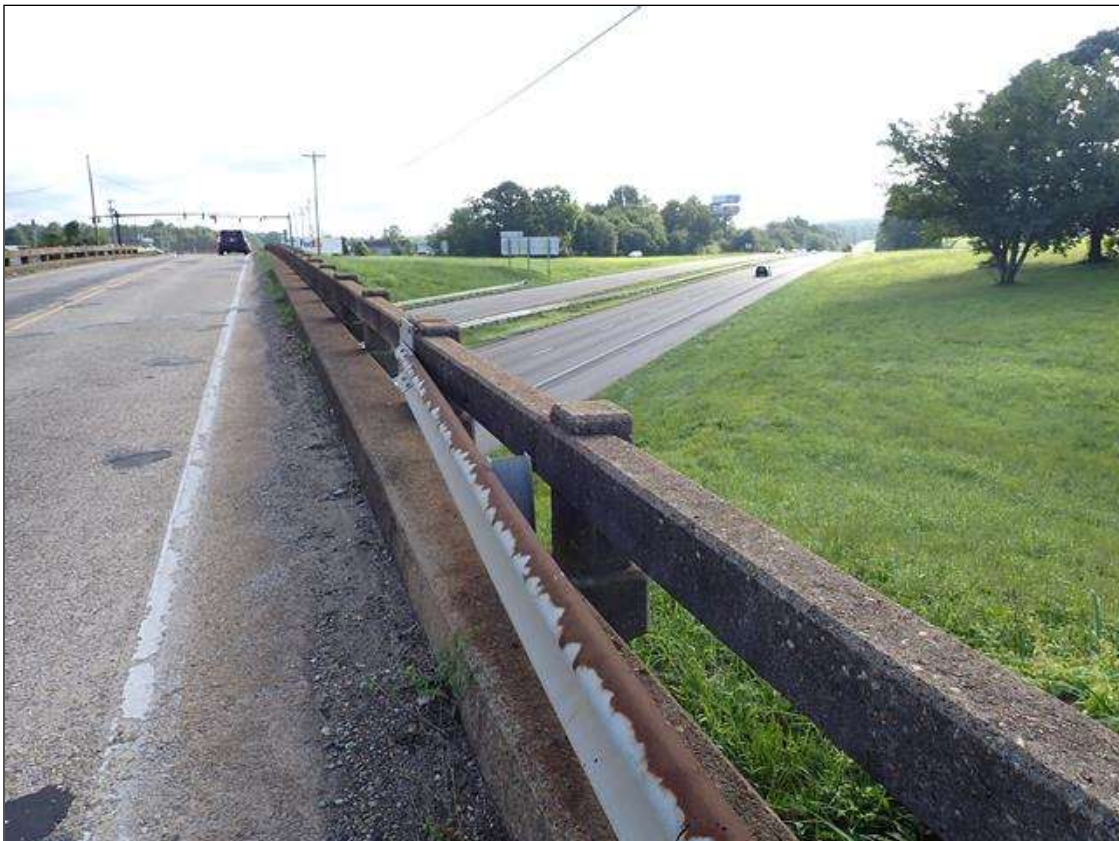
right bridge rail
