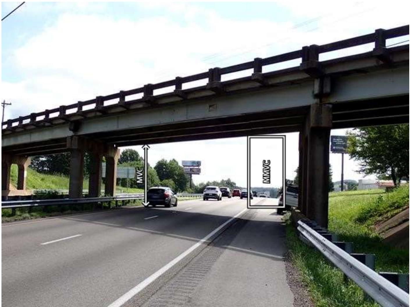
roadway under span 2, looking east (I-40 eastbound)
