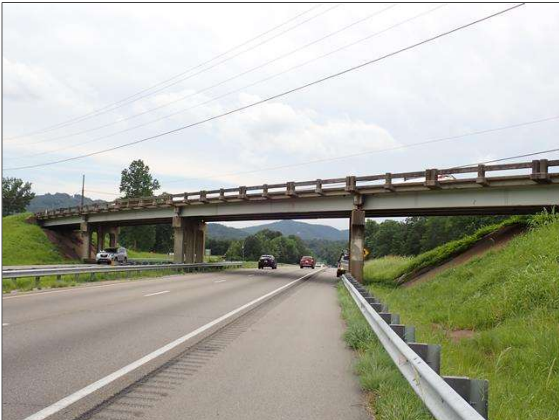
east profile looking west
