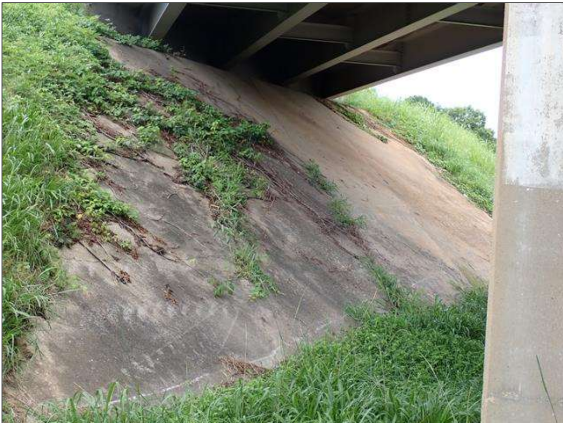
end bent 2 slope protection
