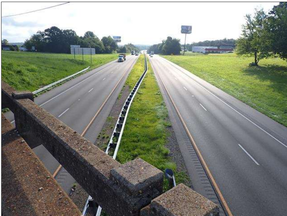
roadway looking east
