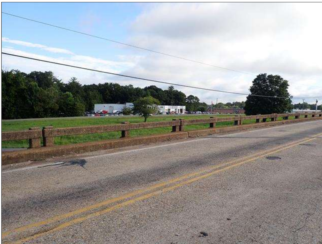
left bridge rail
