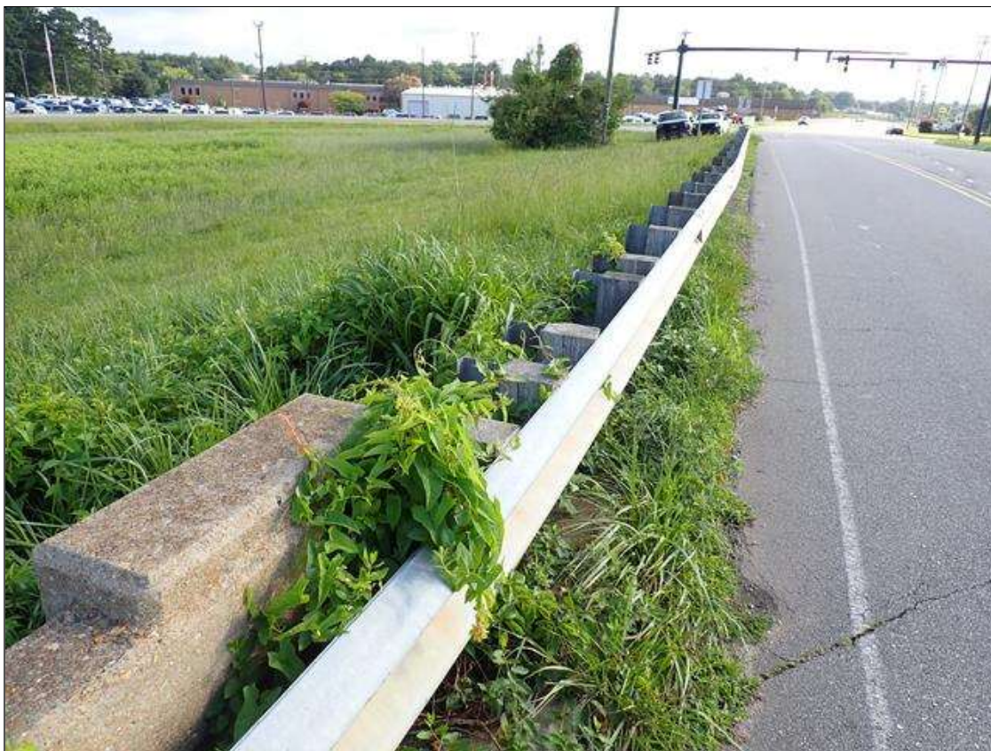
northwest guardrail transition
