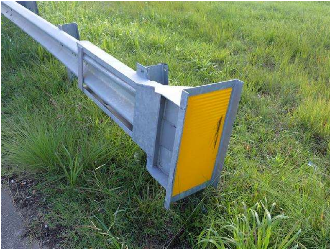
southeast guardrail termination
