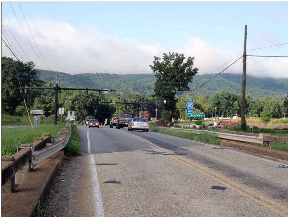
south approach looking south
