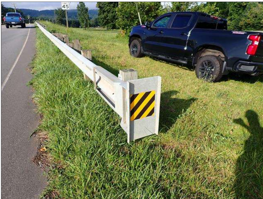
northwest guardrail termination
