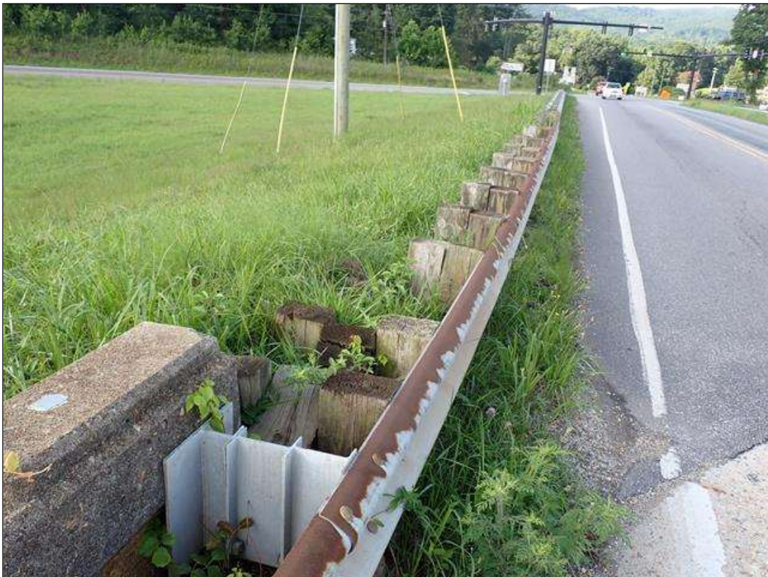
southeast guardrail transition
