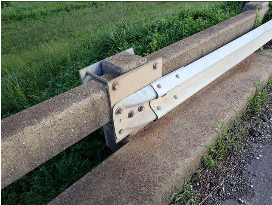
northwest guardrail attachment
