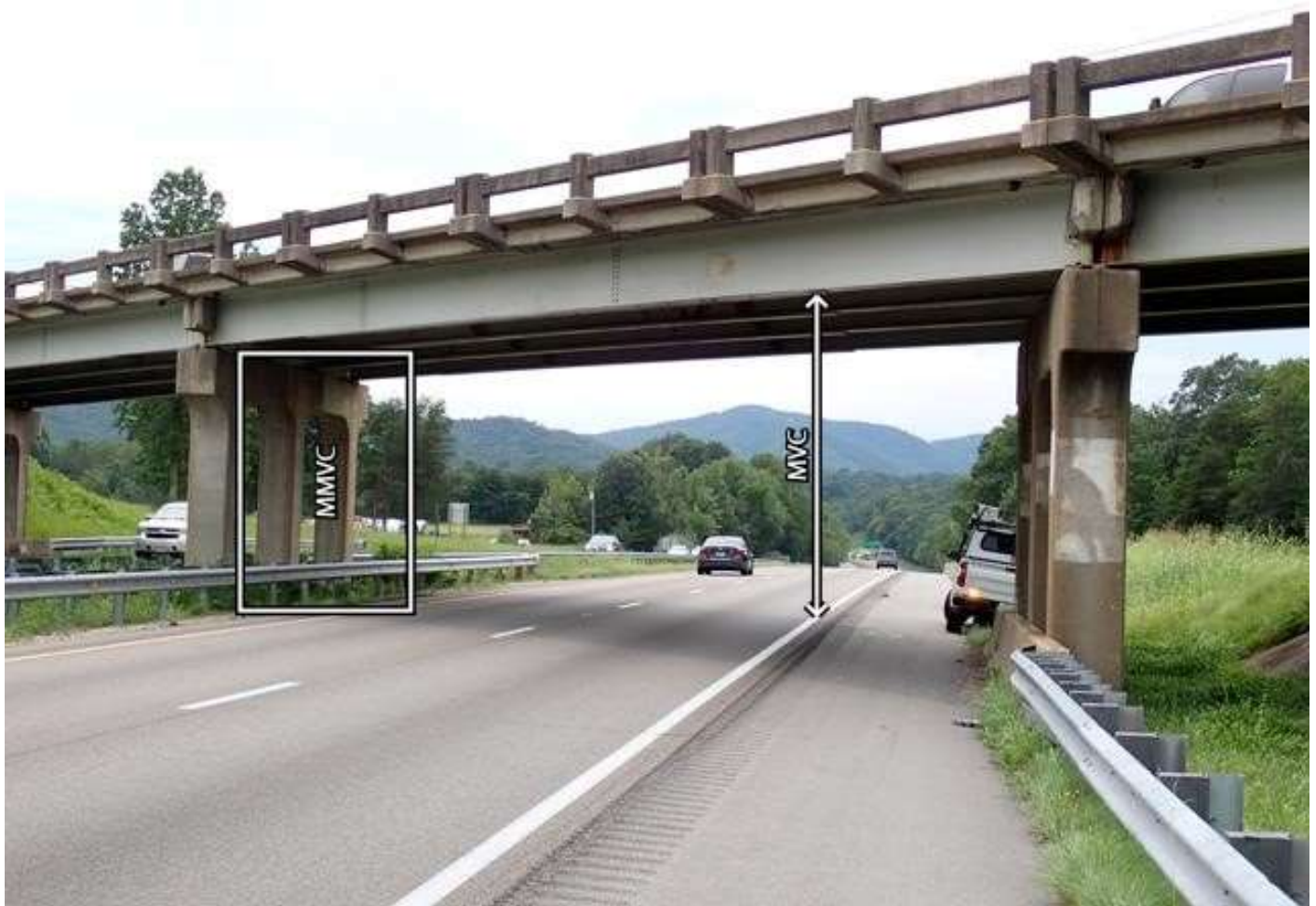
roadway under span 3, looking west (I-40 westbound)
