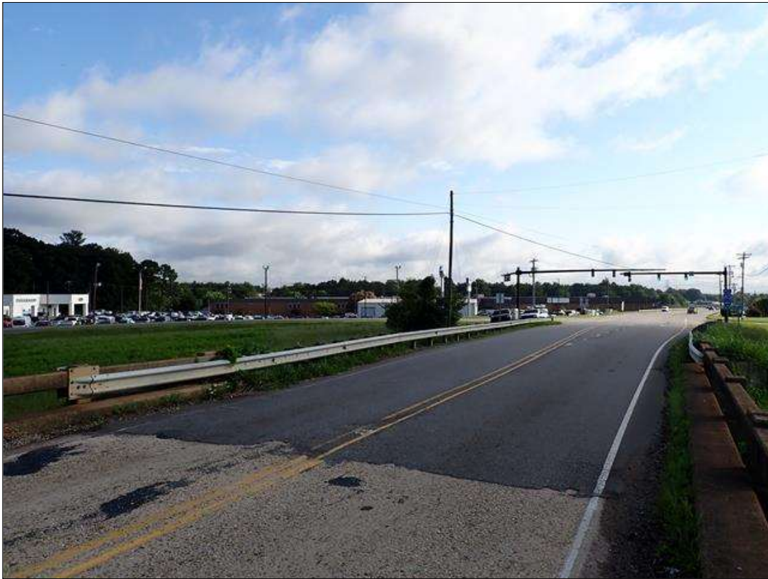
north approach looking north
