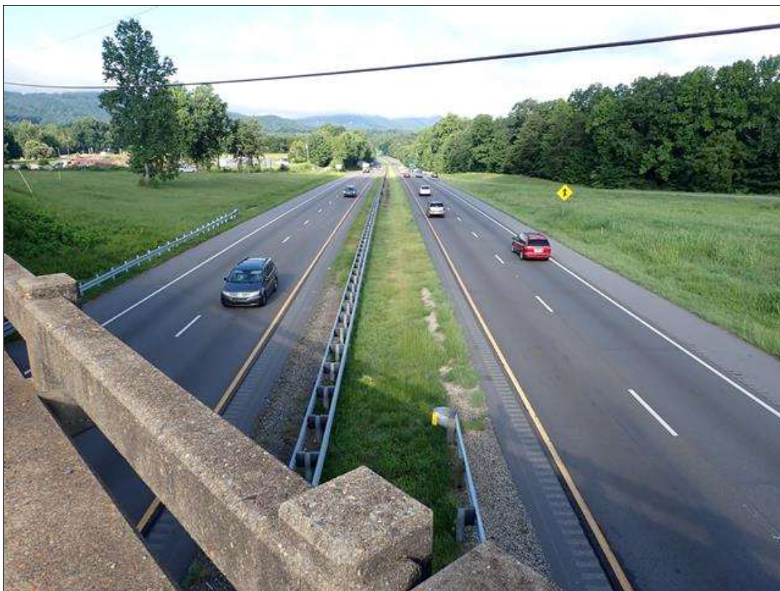
roadway looking west
