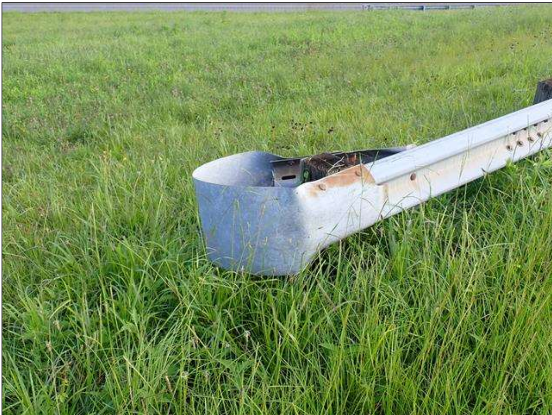
southwest guardrail termination
