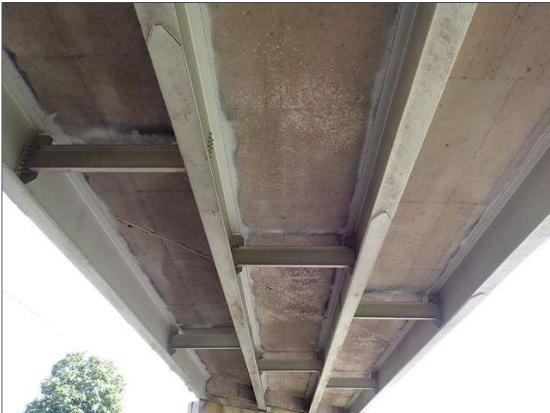
superstructure underside, span 2 (span 3 similar)
