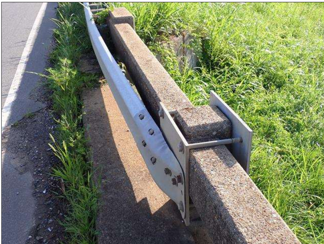
northeast guardrail attachment
