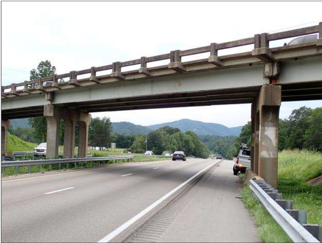
roadway under span 3, looking west (I-40 westbound)
