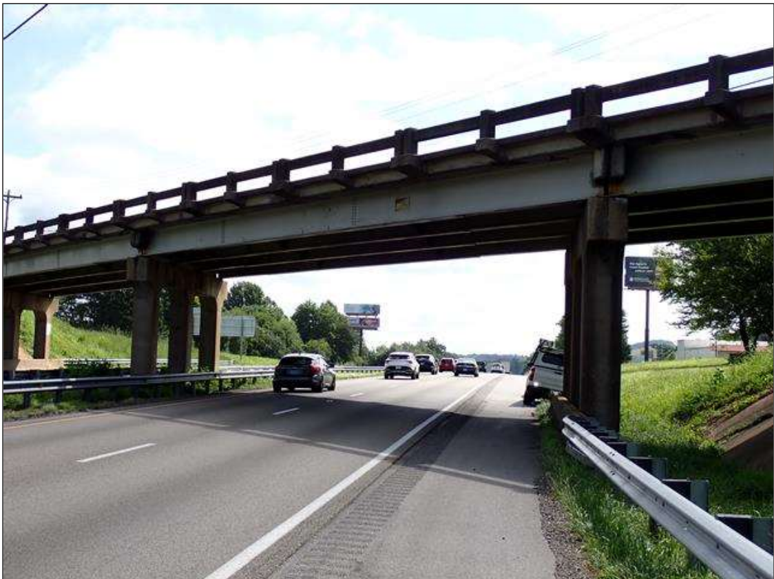
roadway under span 2, looking east (I-40 eastbound)
