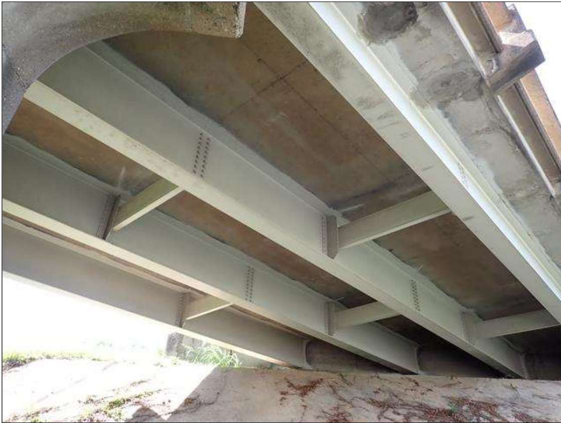
superstructure underside, span 1 (span 4 similar)
