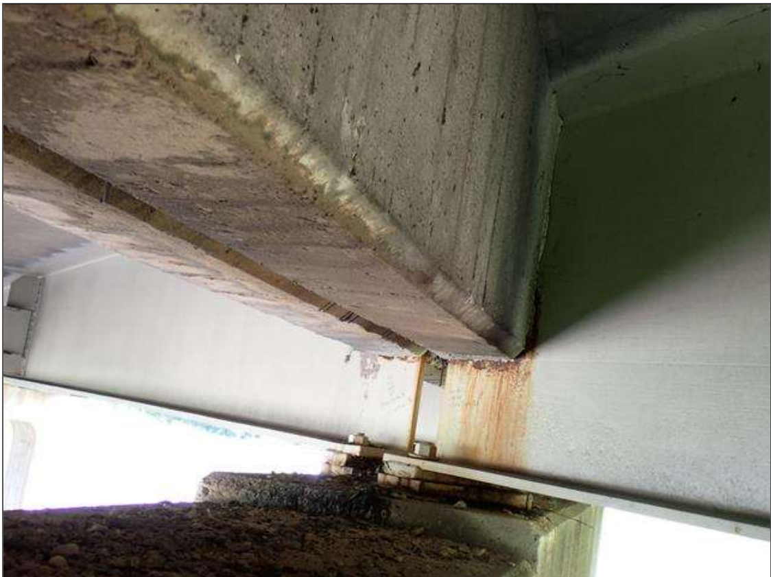
beams over bent
