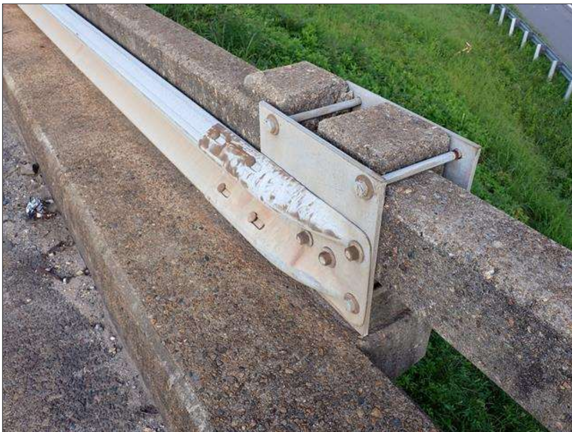
southwest guardrail attachment
