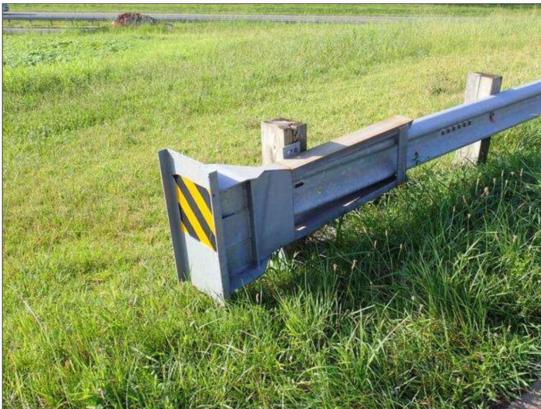
northeast guardrail termination
