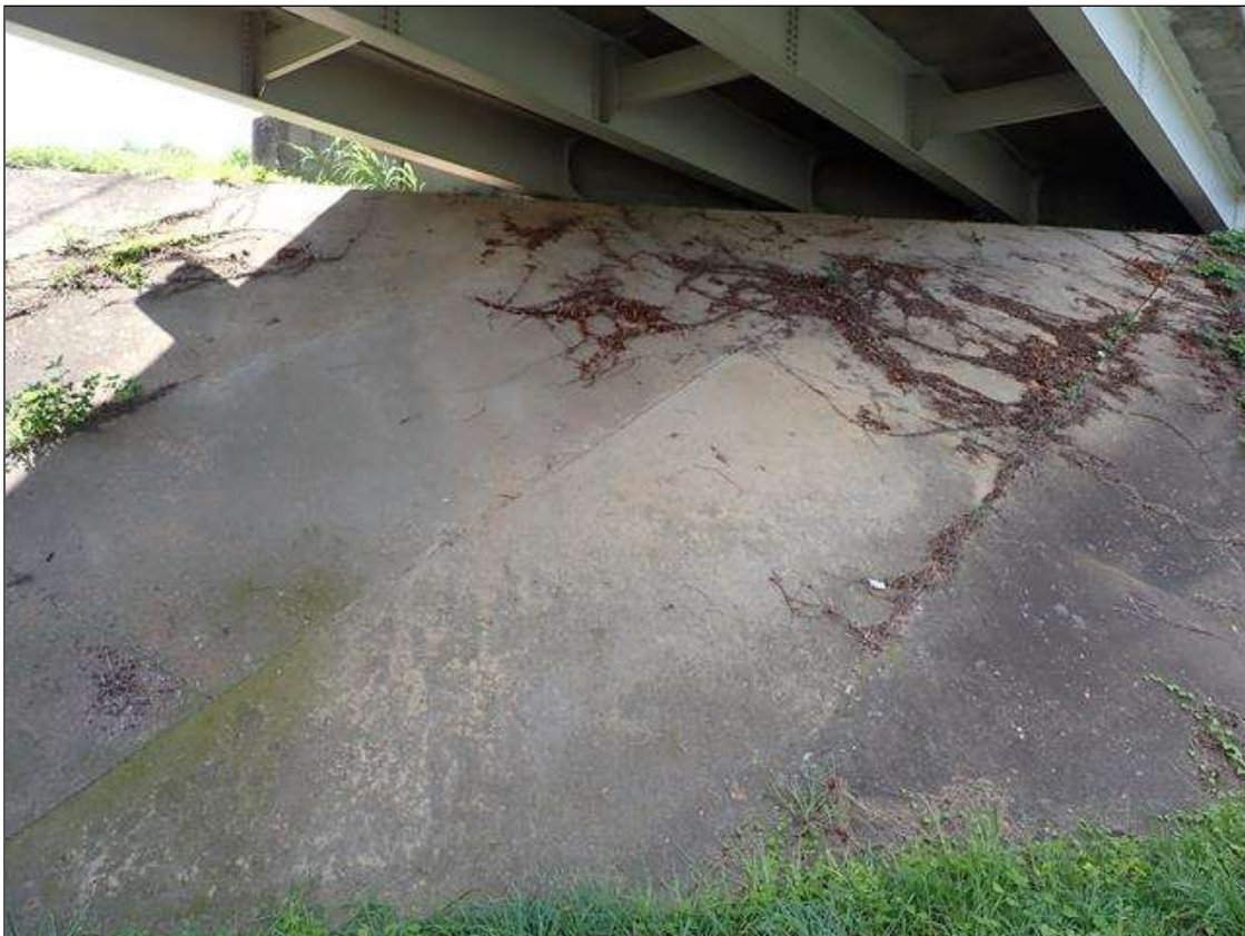
end bent 1 slope protection
